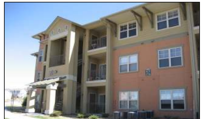
6. View of typical front/side elevation apartment building.
