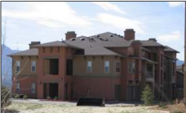
3. View of typical front/side elevation apartment building.
