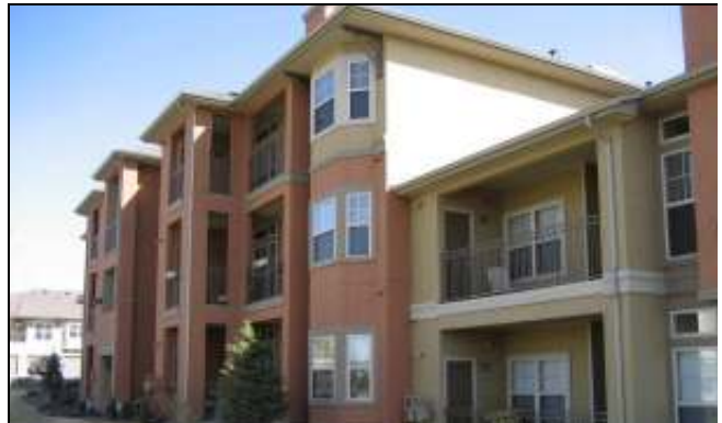
4. View of typical front/side elevation apartment building.
