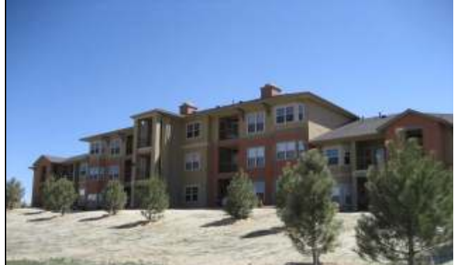
2. View of typical rear elevation apartment building.
