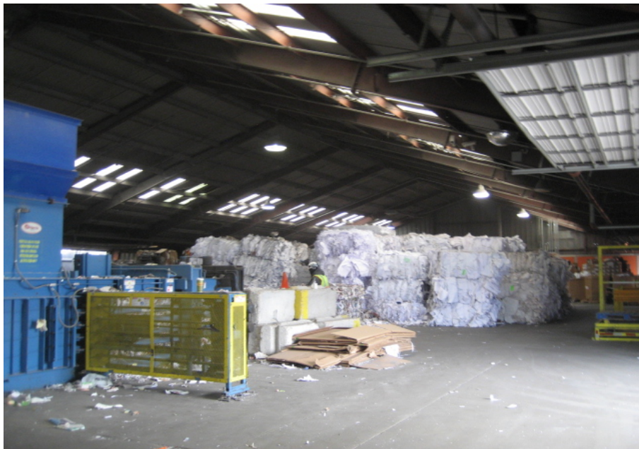
Photograph No. 6 Interior view Building 2
