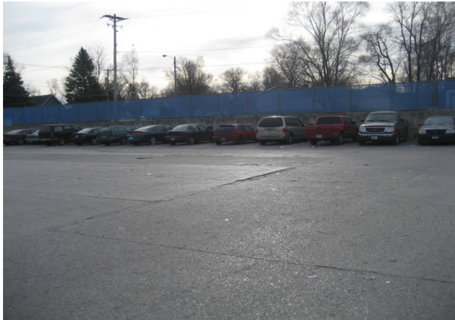
Photograph No. 16 Typical concrete surface parking areas
