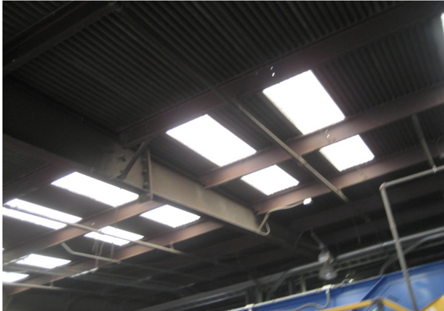
Photograph No. 19 Typical skylights at Building 2
