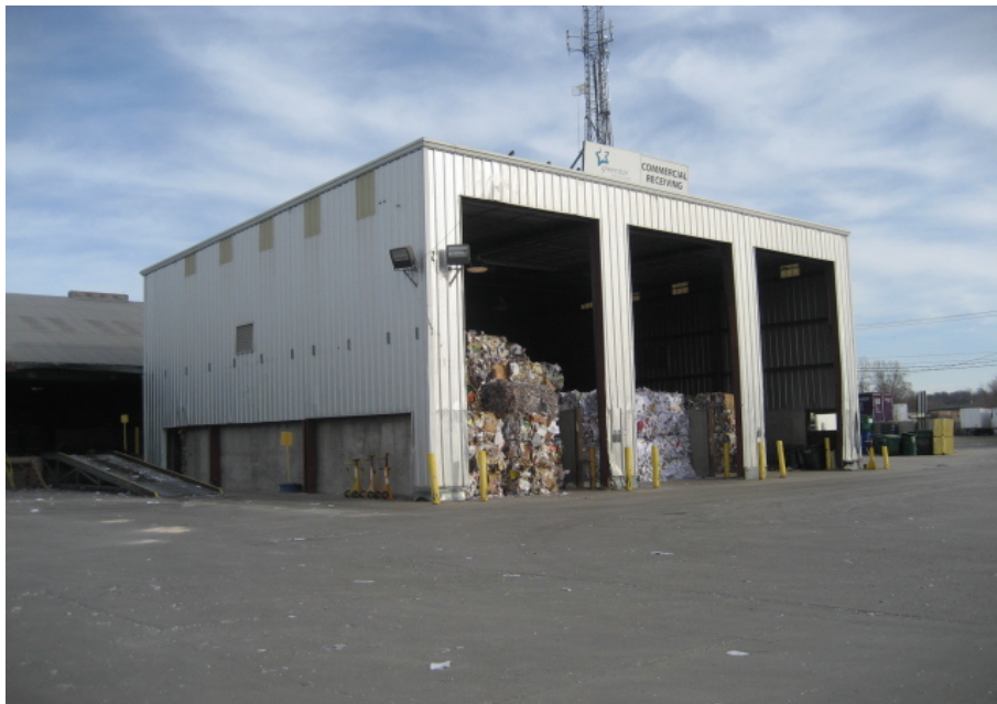
Photograph No. 20 View of typical canopied areas-Building 2
