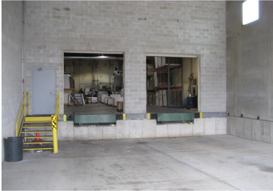
Photograph No. 25 Typical indoor receiving dock area.
