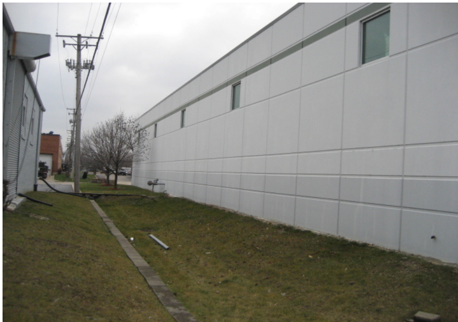
Photograph No. 18 East view of the Property.
