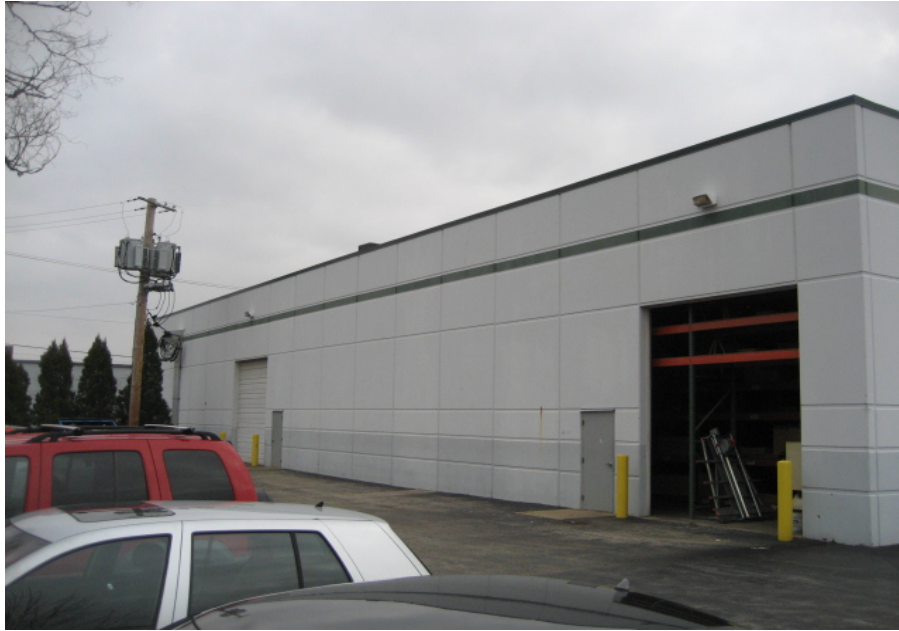
Photograph No. 17 South view of the Property.
