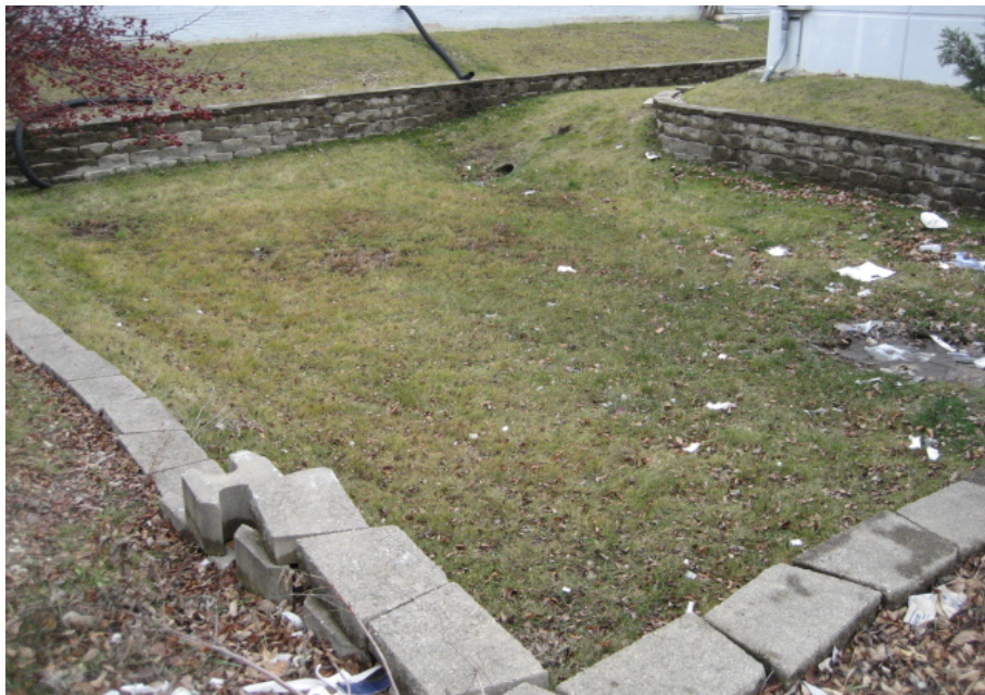
Photograph No. 8 Dry water detention area to the northeast of the Property.
