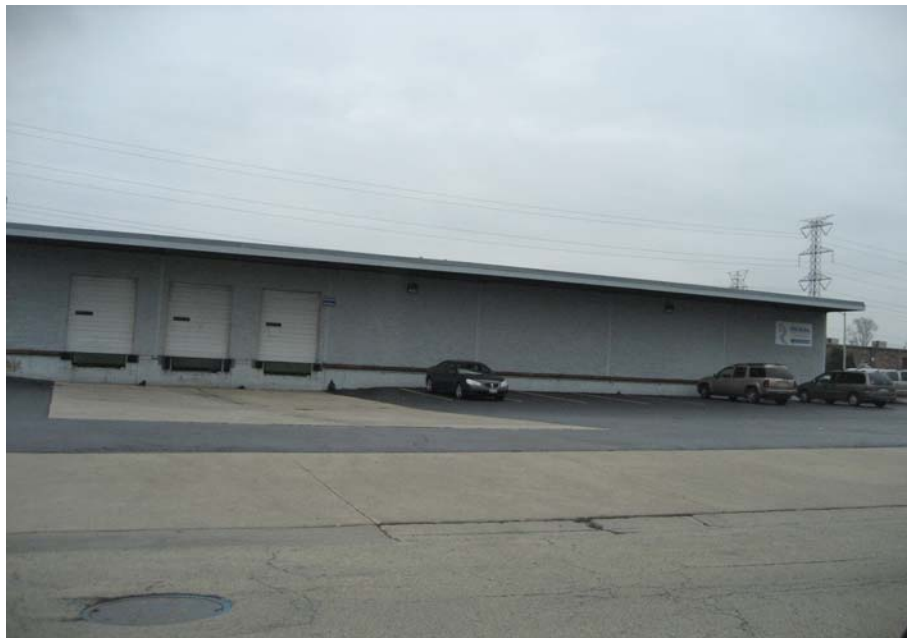
Photograph No. 12 Adjacent Regal Manufacturing Co Inc. east of the Property.
