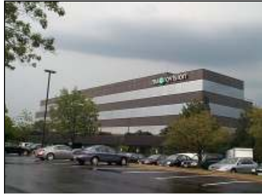
2. South view of building
