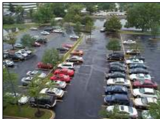
36. Asphalt parking lot
