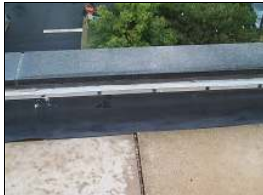
34. Rubber membrane with granite coping on parapet wall
