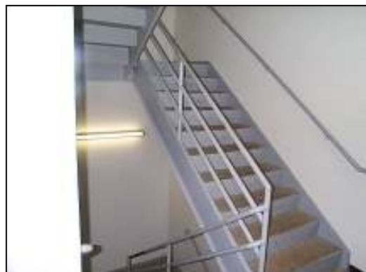
12. Typical stairwell – steel framed with concrete treads and landings
