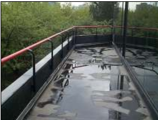
9. Balcony with rubber membrane
