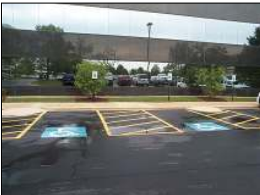
5. ADA parking spaces on south side of building
