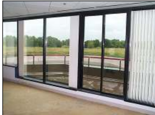
8. Sliding glass doors lead to each balcony
