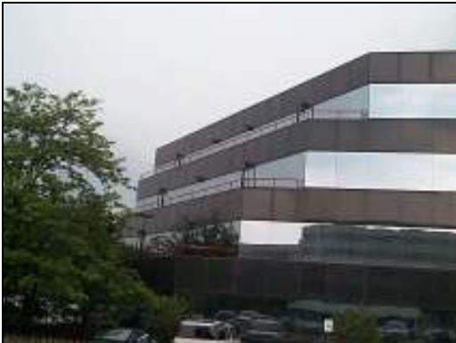
7. Balconies on both the west and east sides of the building (floors 2-4 only)
