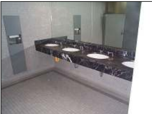
15. Common area bathroom sinks – 1 ADA compliant (yellow trap pad)
