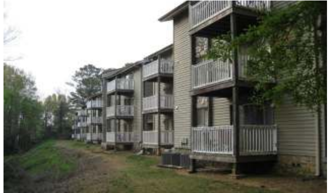
2. View of typical rear elevation apartment building.
