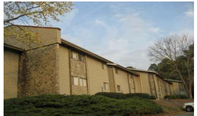
4. View of typical front/side elevation apartment building.
