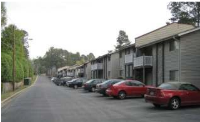
3. View of typical front/side elevation apartment building.
