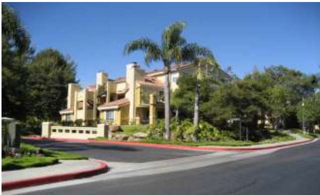
3. View of typical front/side elevation apartment building.
