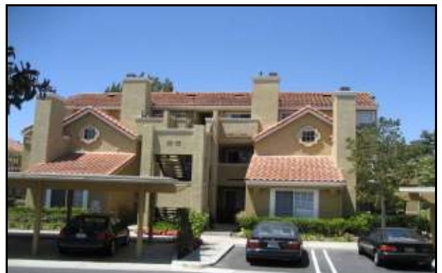
6. View of typical front/side elevation apartment building.
