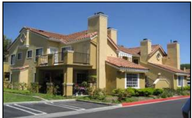
4. View of typical front/side elevation apartment building.
