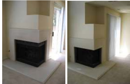
20. View of typical fireplace.
