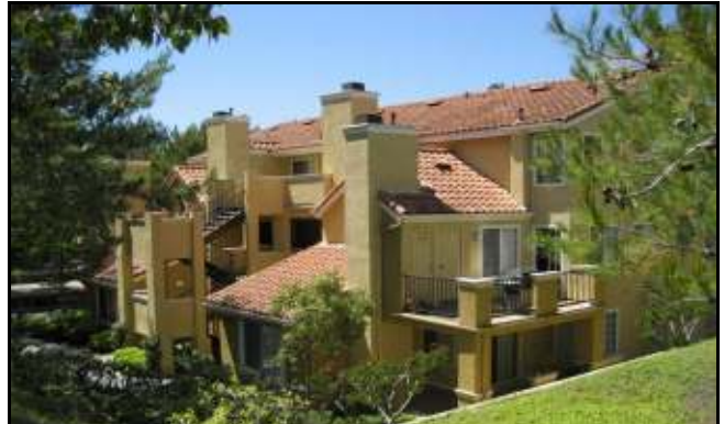
2. View of typical rear elevation apartment building.
