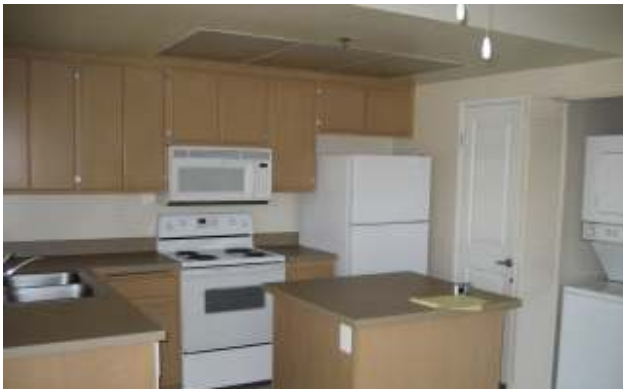
7. View of typical kitchen area.
