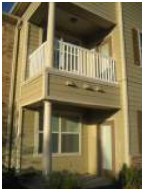
9. PVC RAILINGS AT UPPER LEVEL PATIOS
