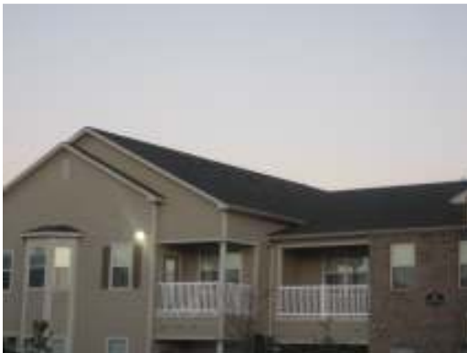
21. ASPHALT SHINGLE ROOFING
