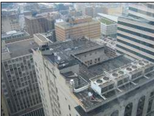
5. SOUTH VIEW (ROOF TOP)
